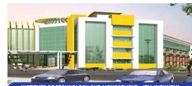
INSTITUTE OF TECHNOLOGY AND MANAGEMENT - ITM LUCKNOW
